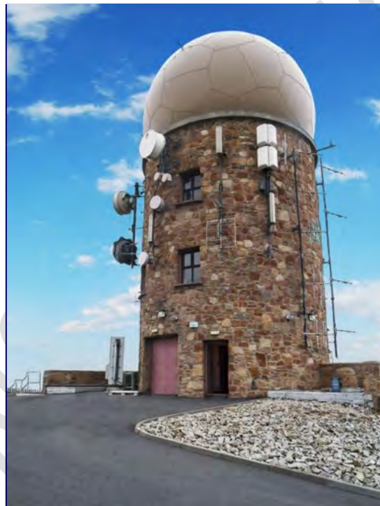
Figure 2 - Monopulse Secondary Surveillance Radar (MSSR) Installation at Dooncarton, Co. Mayo
