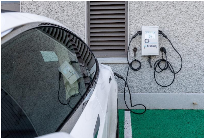
Figure 17: EV charging point in IAA Ballygirreen
