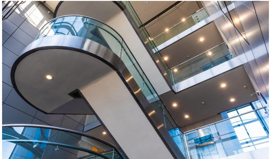
Figure 12: LED lighting installation
