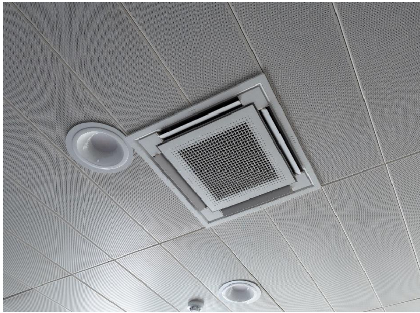
Figure 10: New VRF heating and cooling system and new LED lighting installation at IAA facility
