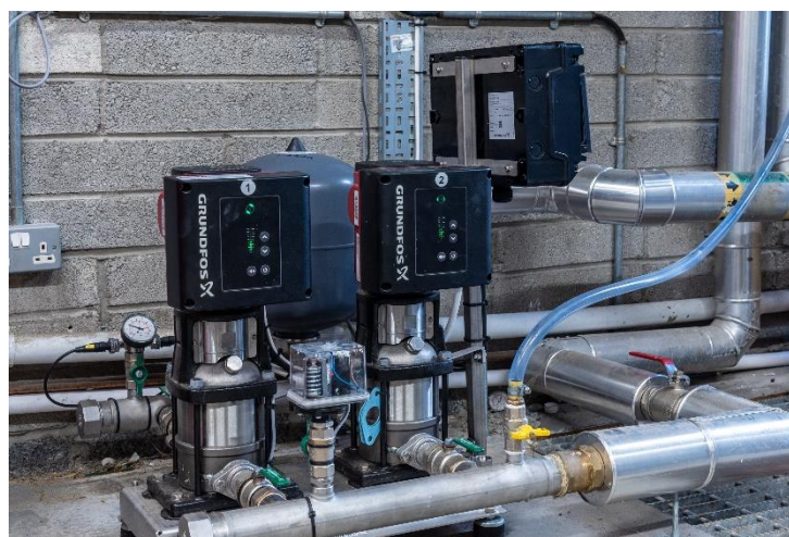
Figure 9: New high efficiency service pumps installation at IAA facility
