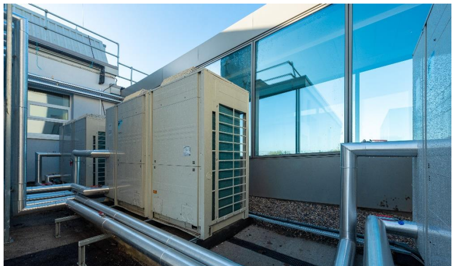
Figure 13: VRF heat recovery system installed in IAA Shannon Centre in Ballycasey
