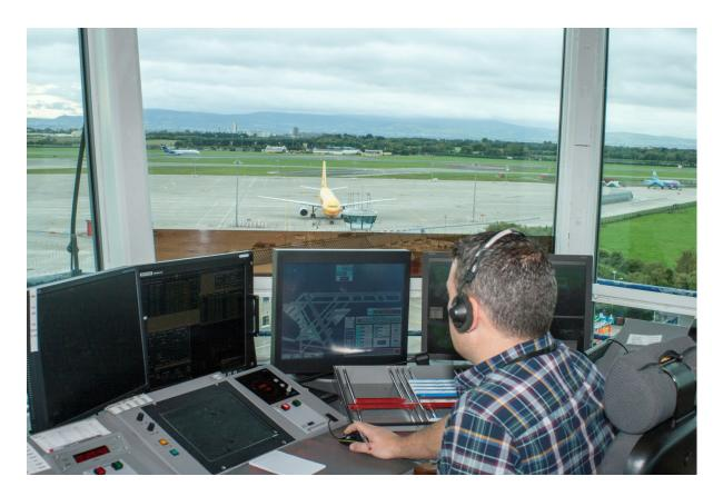
This photo shows the Air Movements Controller's working position. The ATC Eurocat workstation consists of the two screens on the left of the picture, which display radar data as well as ancillary information such as flight plan data or weather information. At lower left is the communications control panel, and to its right is a board for managing flight strips. The screens to the right are used for controlling airfield lighting and the airfield surface movements radar system.
