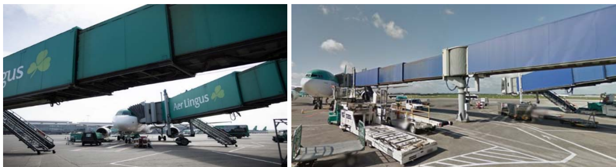
Figure 1 3 tunnel section airbridges used in Pier 4 & Pier 3
