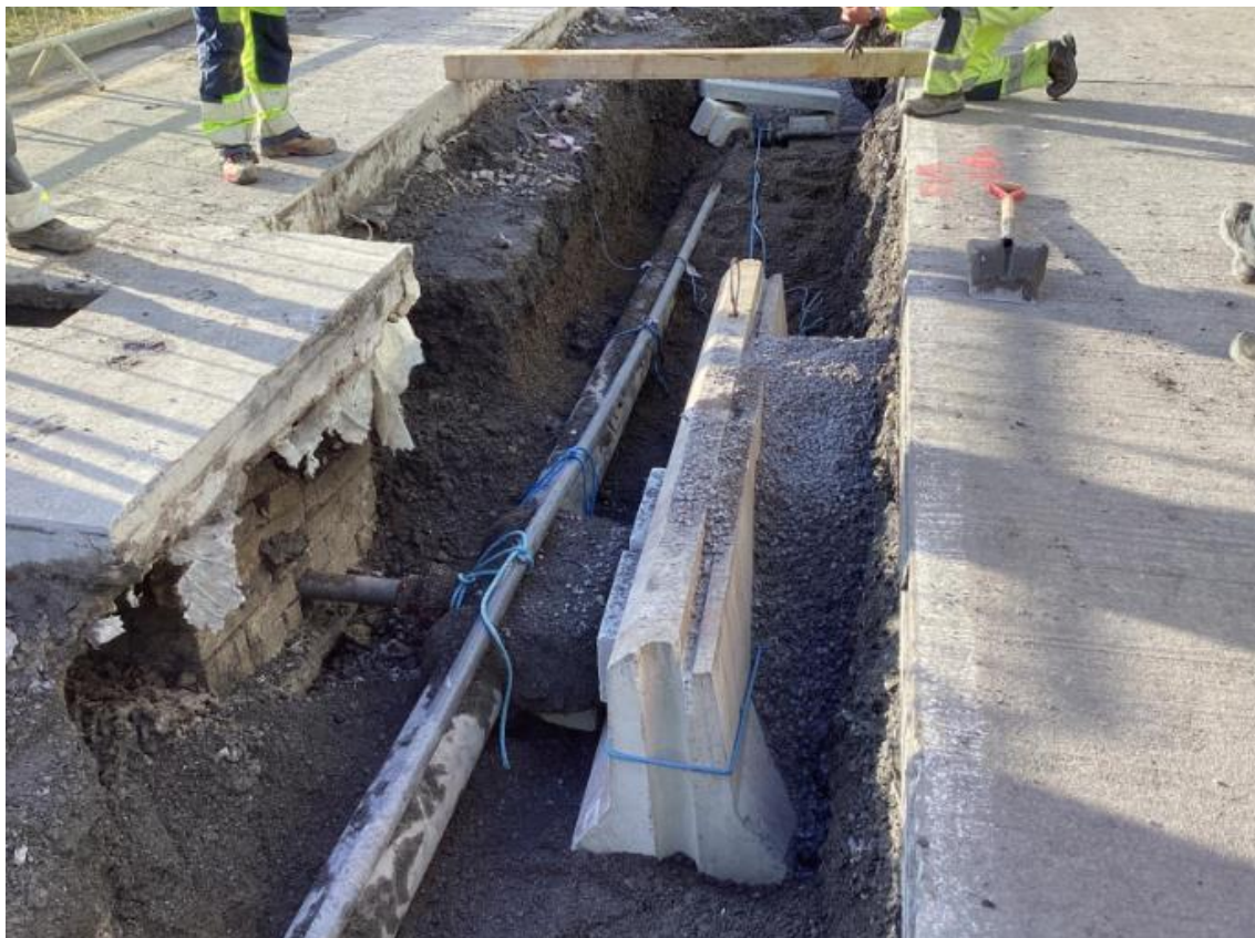
Figure 6.18: CIP27.04.22 – Potable and Foul Water Upgrades - Installation of Resilience Route for Reservoir to Airport Ring Trunk Main
