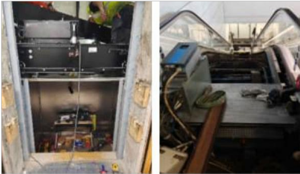
Figure 6.17 Example of Terminal Lifts and Escalators Modernisation Works
