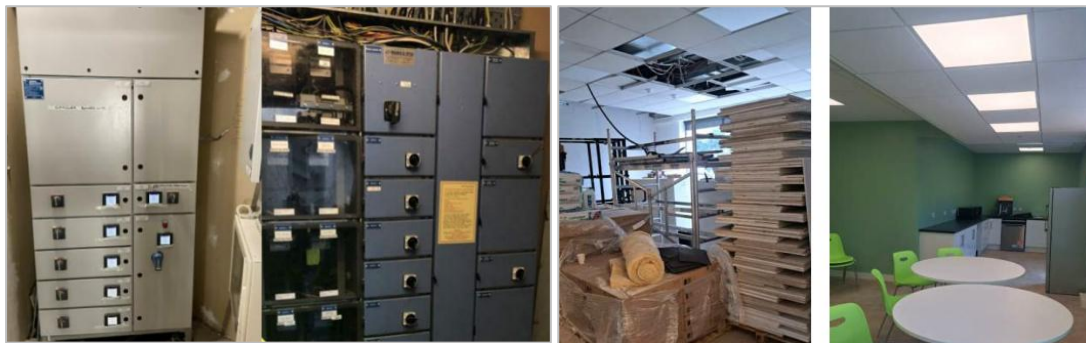
Figure 6.16: CIP27.04.19 Campus Buildings M&E and Life Safety Systems - Local Sub Main Electrical distribution Replacement, Refurbishment of Services in Campus Building and LED upgrade installation
