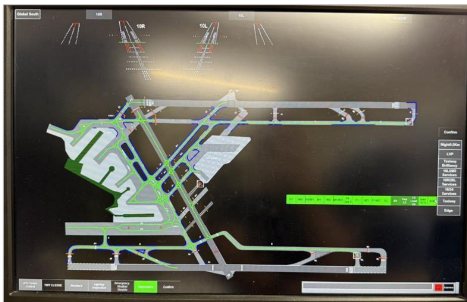
Figure 6.7: CIP27.04.06 – Airfield AGL Substation Improvement Programme - AGL Controls Screen
