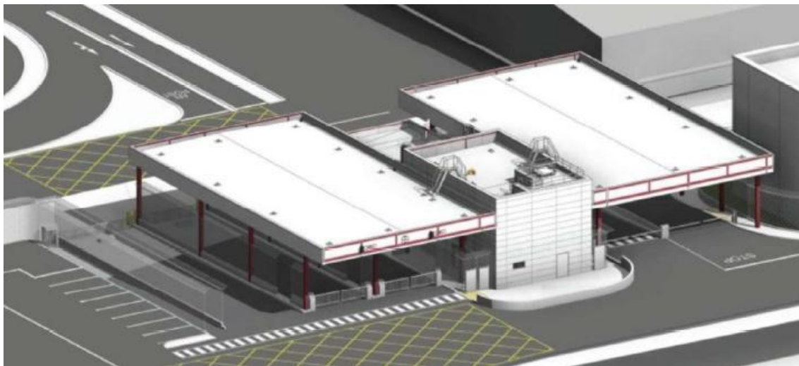
Figure 4.7: CIP27.02.07 – Gate Post 4 Relocation Overview
