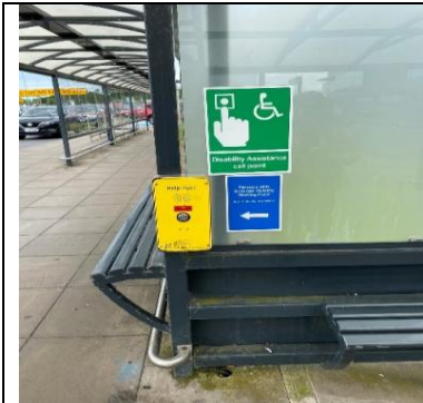
Figure 1 PRM Call Point located in walkway outside terminal building
