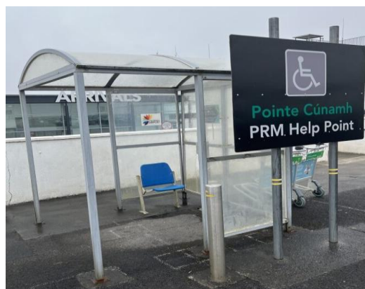
Figure 2 PRM seating at exterior call point
