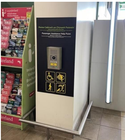
Figure 4 PRM call point at Terminal 1
