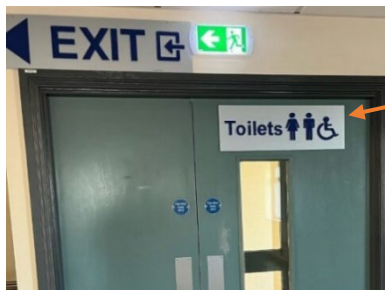
Figure 8: Sign indicating accessible bathroom (bathroom is not accessible)
