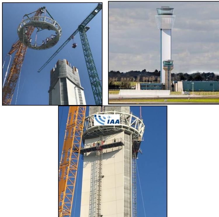
Figure H.2: Progress on Control Tower at Dublin Airport
