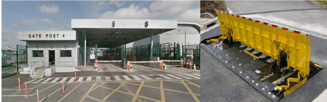
Figure 9.6: Surface Road Blockers & Temporary Mobile Barriers
