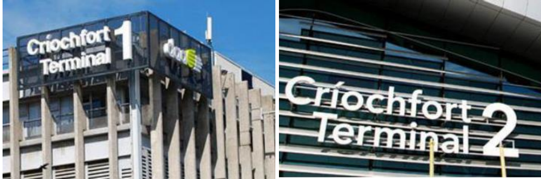
Figure 4.17: Piers and Terminals Critical Maintenance
