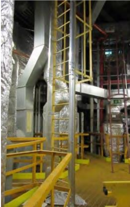
Figure 5.9: Pier 3 Life Extension Works - Mech, Elec & Foul Drainage
