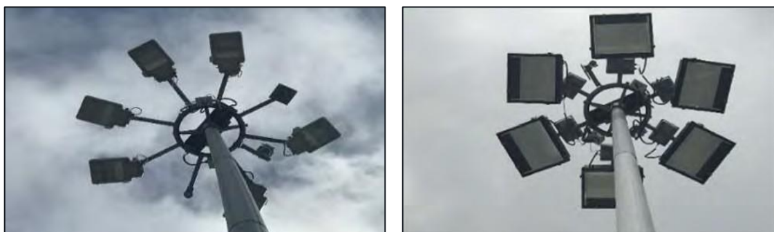
Figure 4.11: High Mast Lighting Improvement
