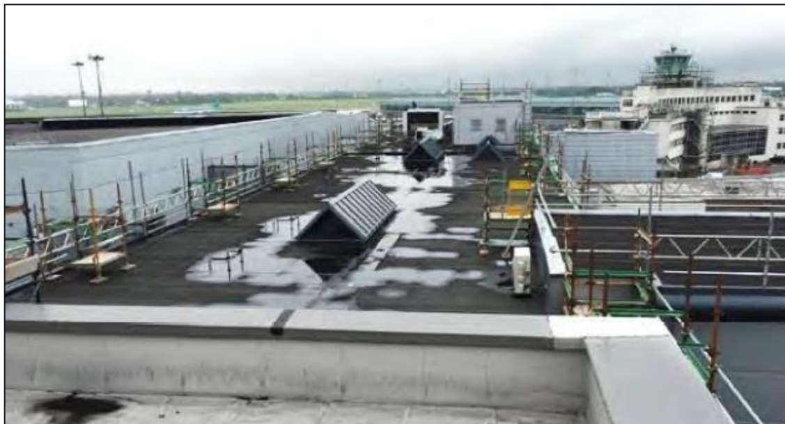
Figure 4.16: Terminal 1 Storm Water Drainage System - T1 Roof
