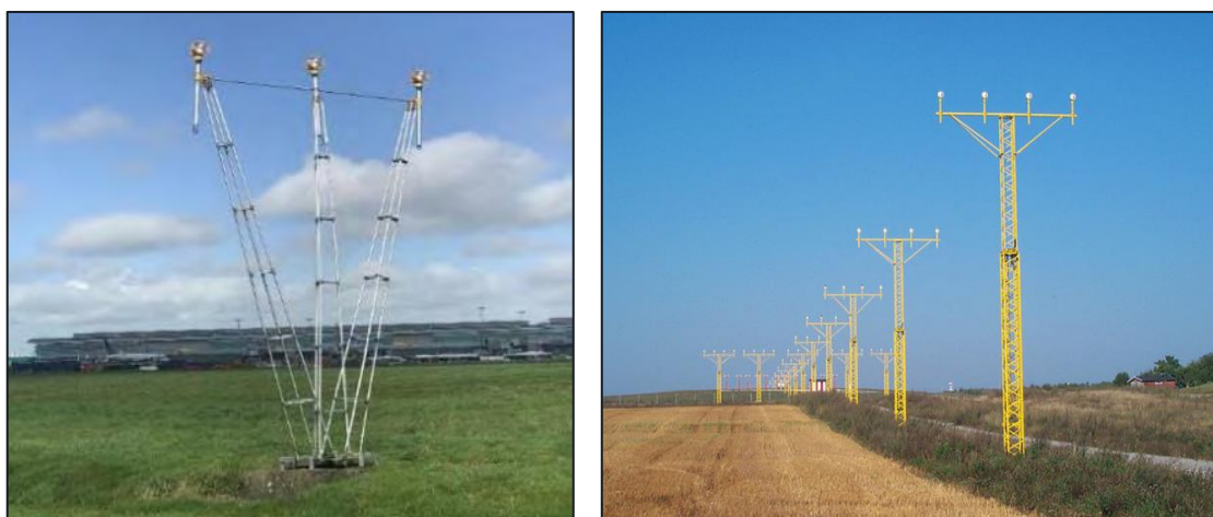
Figure 4.6: Runway Approach Lighting Mast Improvement Programme - (Existing left, typical proposed right)
