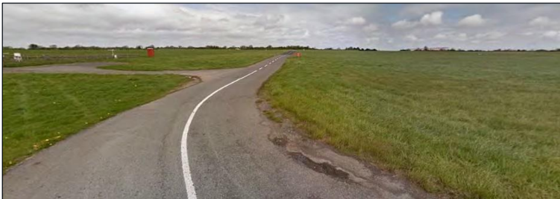
Figure 4.5: Airfield Southern Perimeter Road Upgrade Programme
