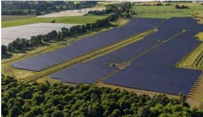
Figure 5.11: Large Energy Project – Photovoltaic Farm
