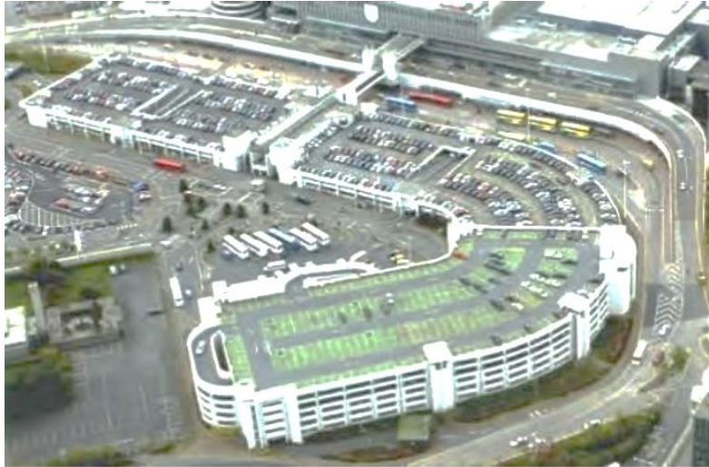
Figure 7.7: Terminal 1 Multi-Storey Car Park Block B
