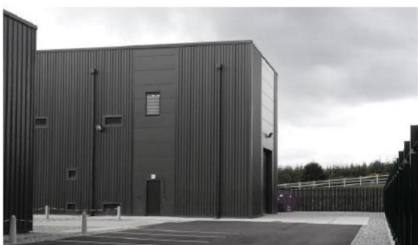
Exhibit 6.16 – Typical ESB GIS Substation
