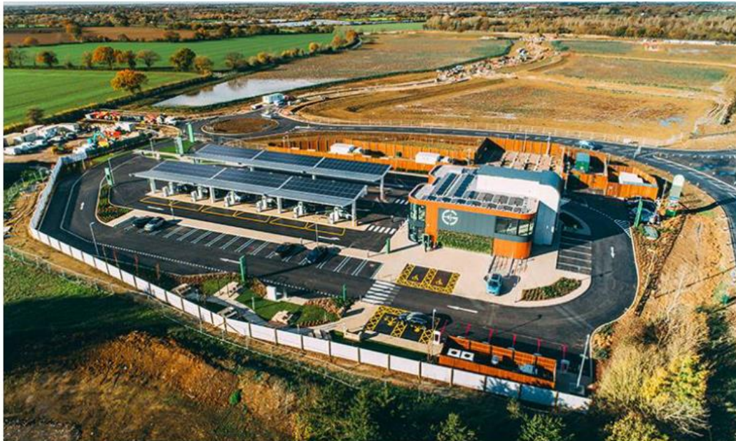
Figure 7.2: Airport EV charging
