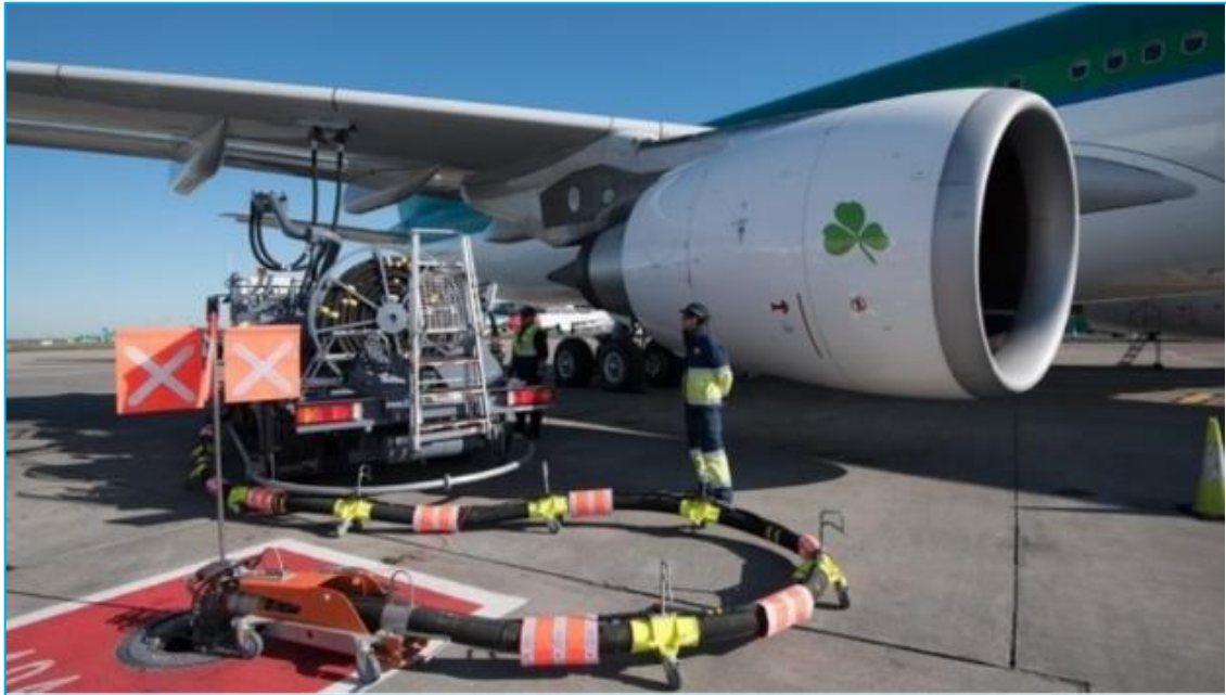
Figure 5.21: Fuel Hydrant Network
