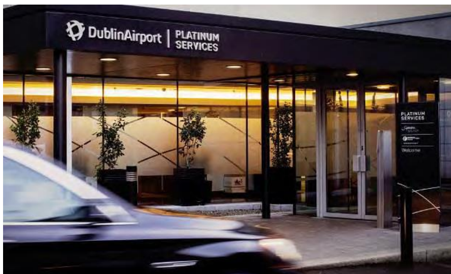
Figure 6.10: Platinum Services Upgrade Works
