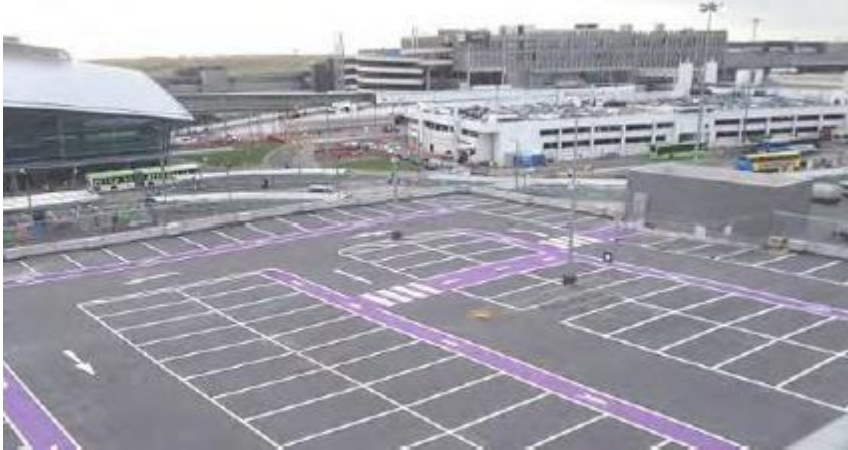
Figure 6.7: Terminal 2 Multi-Storey Car Park
