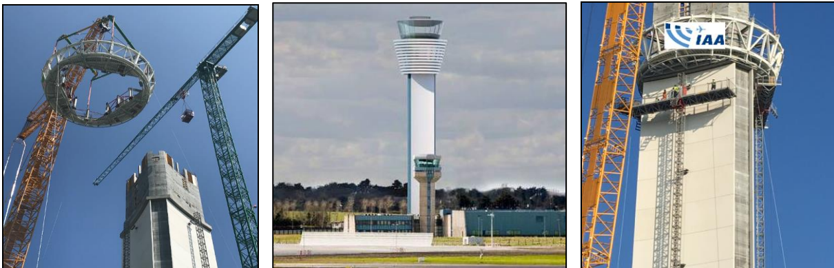
Figure 16 Progress on Control Tower at Dublin Airport
