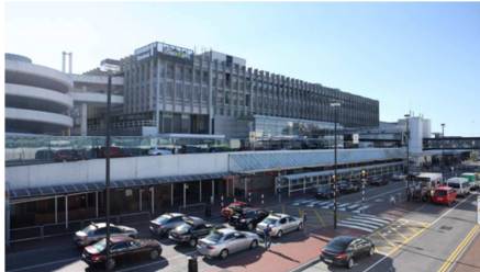
Terminal 1 façade remains as it is now
