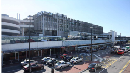
Terminal 1 façade remains as it is now
