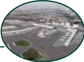
COPENHAGEN €BN 2.6 New Piers & Terminal expansion
