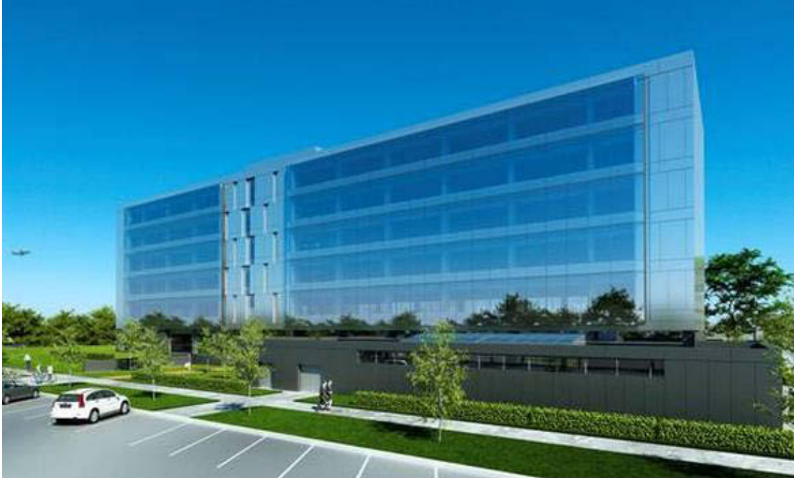
Fig. 6 - Photomontage of the proposed refurbished Aer Lingus Building under Reg. Ref. F14A/0436
