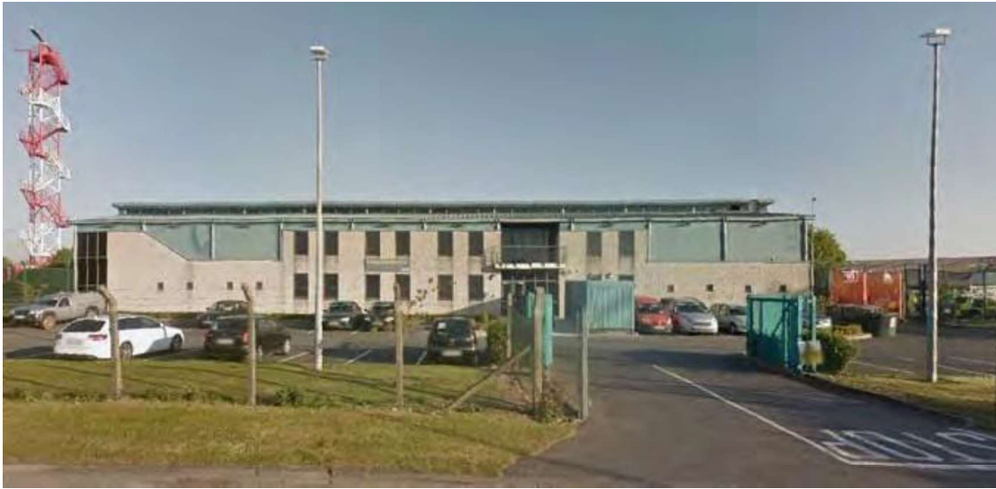
Exhibit 2.3 – Existing Airfield Maintenance Base
